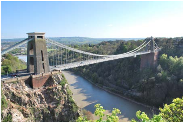
Avon Gorge Suspension Bridge showing the Carboniferous Limestone supporting the piers
