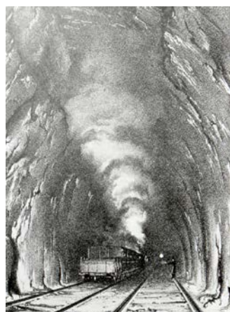
The unlined interior of the tunnel lithograph by J C Bourne
